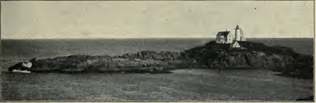
FIG. 67. — A lighthouse built on a small island at the tip of a cape.
